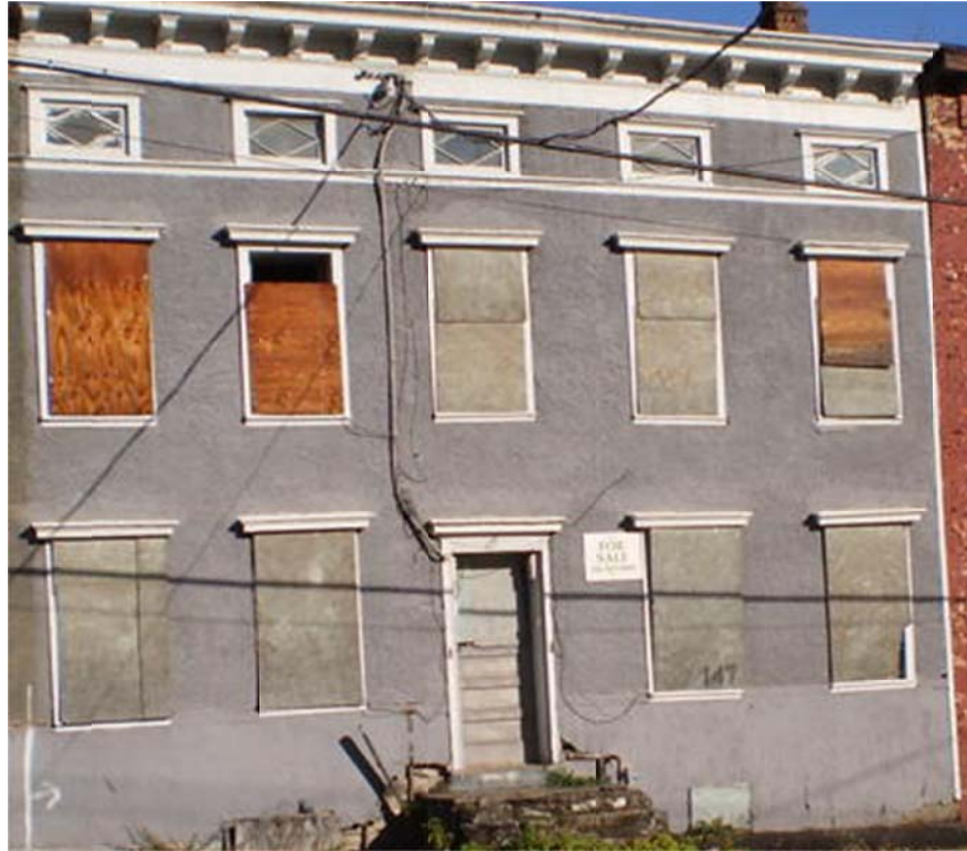
Figure 9: Substantially Deteriorated Example
